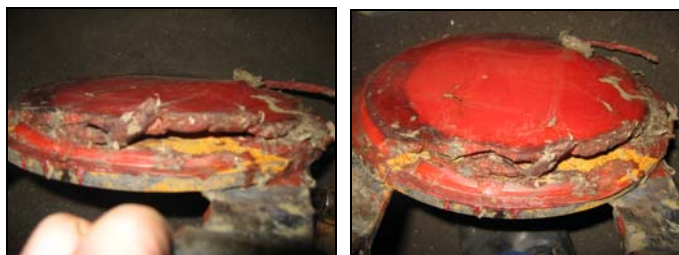
Existing worn coating
