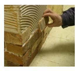
Portland cement and aggregate, but the mason's mortar will have a courser grind to the aggregate, which can give the installation a more authentic brick look. Some people will choose to use a sanded tile grout, especially if they are trying to get a specific color.
