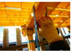
NOTE: A minimum of 2 cam straps should be used to tie down every overlapping panel.
