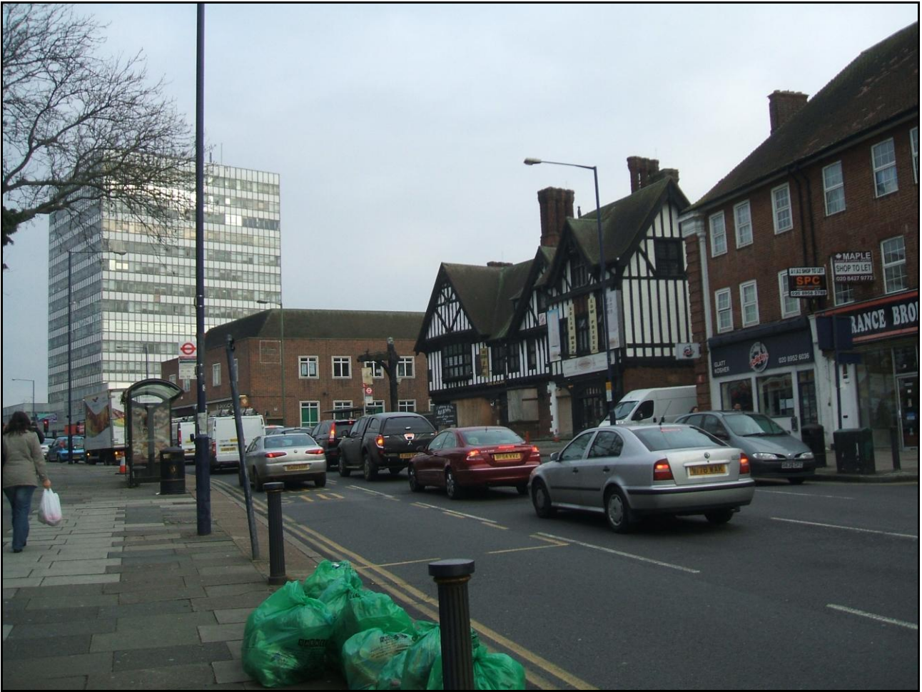
The Green Shield Stamp building (now Premier House) towering over older Station Road buildings, including the boarded-up-and-soon-to-be-demolished mock-Tudor Railway Hotel
