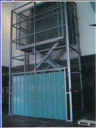
● SCISSORS GOODS LIFTING PLATFORM AT SENOKO
