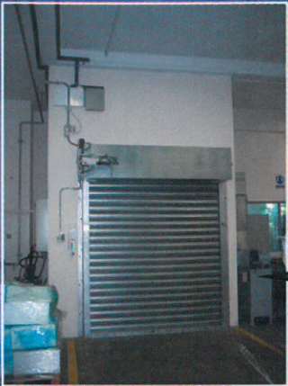
● GOODS LIFTER AT CHANGI NORTH FACTORY
