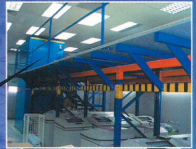
● SAMPLE VERTICAL GOODS LIFT FOR MEZZANINE FLOOR
