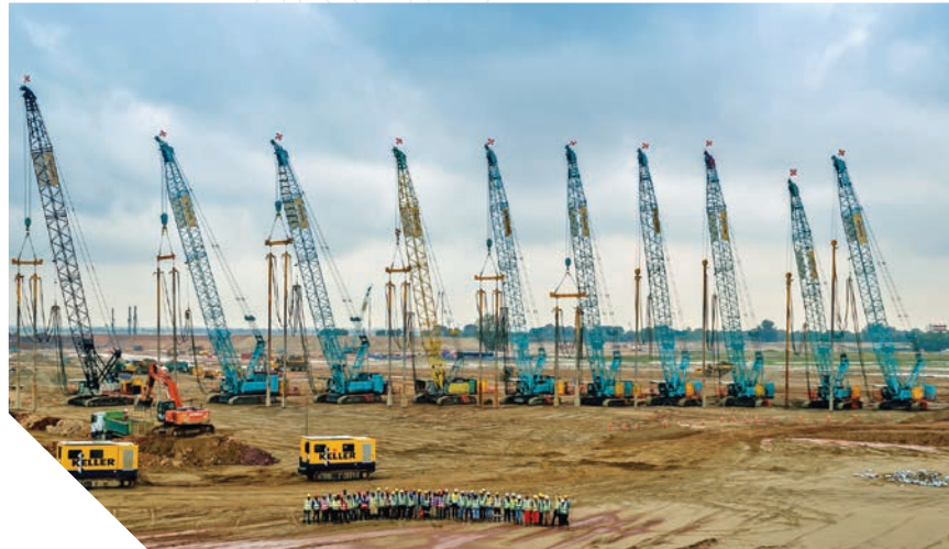
Vibro Compaction works for an airfield development, Singapore
