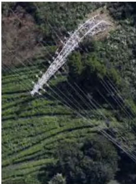
Transmission tower collapsed in Chiba Prefecture
