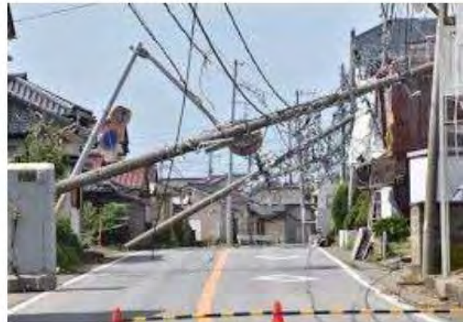
About 2,000 Electric poles collapsed in Chiba Prefecture
