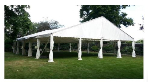
The Clearspan Marquee is exactly as the name suggests – with no internal poles you have the advantage of being able to use all of the internal floor space.
