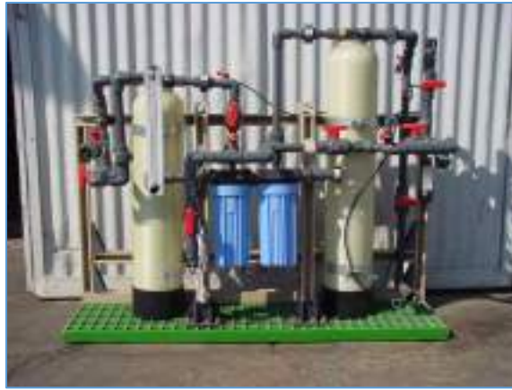
Typical Carbon & Mixed Bed Ion Exchange Arrangement.
