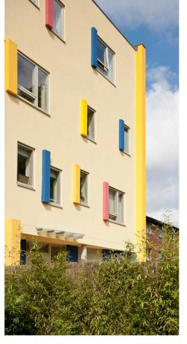
The project involved the demolition of the existing building and the construction of the seven new homes over four storeys. Traditional load bearing block work with precast floors was used in the build. New vehicular access was created, along with five car parking spaces to the front of the site, a bicycle store and refuse/recycling store. The building was finished with multi-coloured facade detailing and high quality landscaping.
