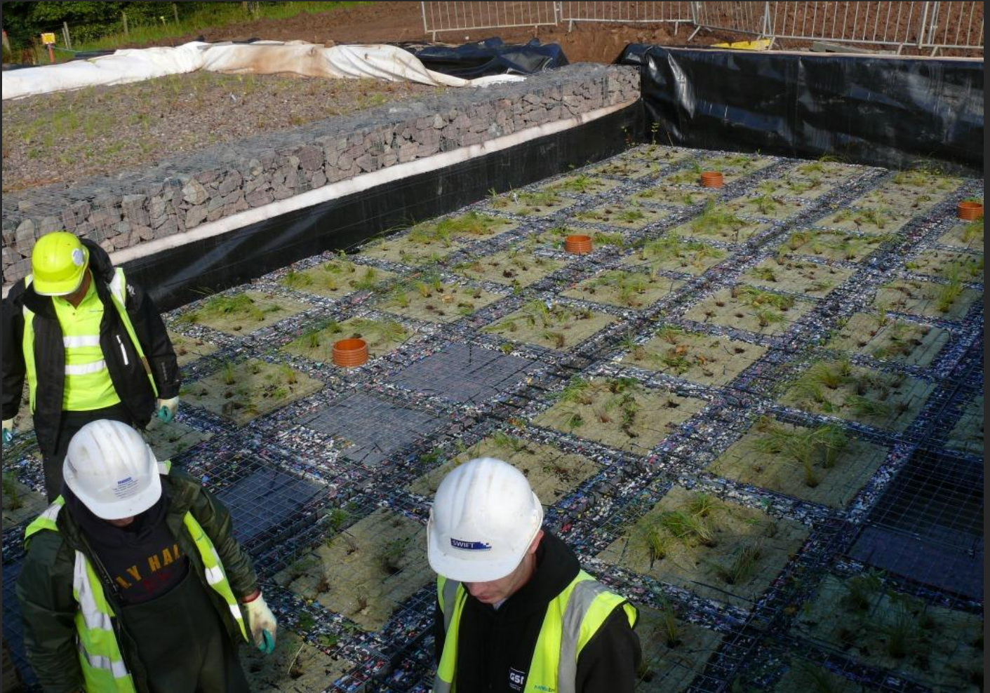
Scottish Water, Carlland Low Carbon STW – Installation of Floating Reedraft Cover
