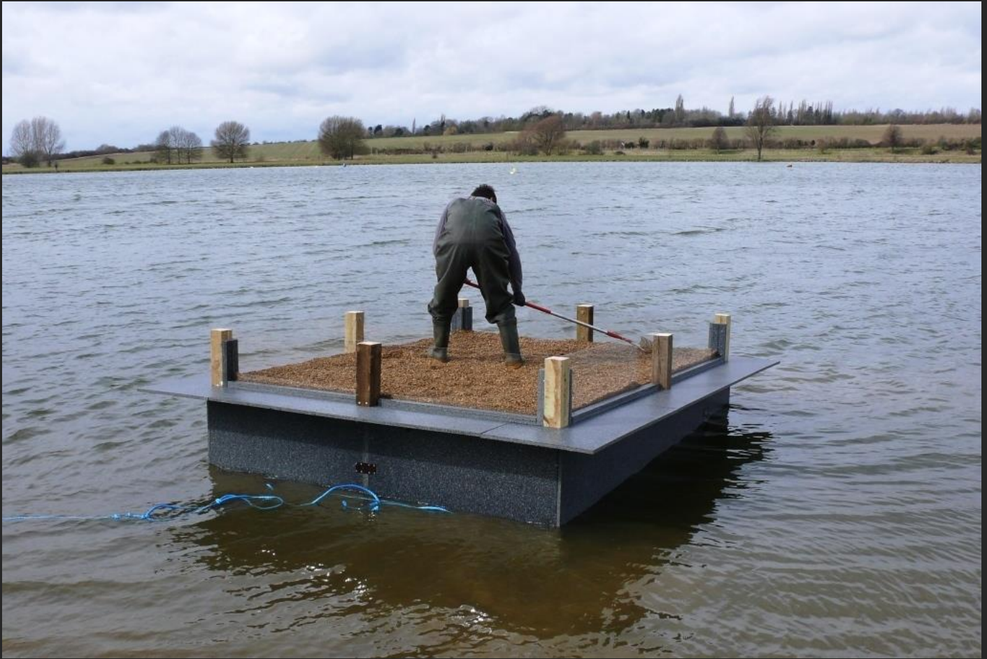
2 tern nesting rafts designed to be both mink and otter proof, with Perspex sides for 'birders' – installation at the Nene Park Trust Peterborough March 2013.
