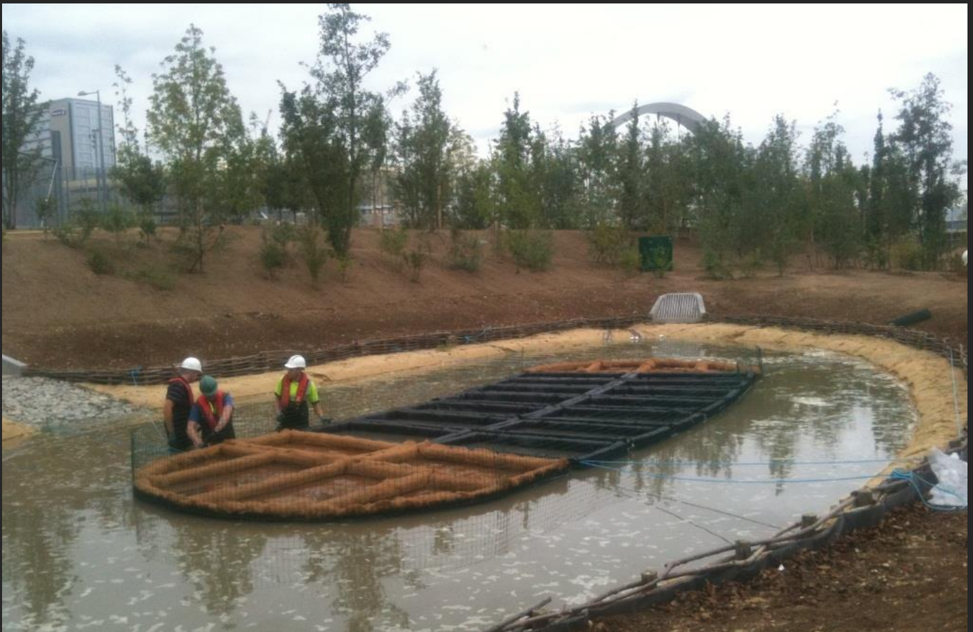
Floating reedrafts designed, fabricated and installed at the 2012 Olympic Constructed Wetlands.
