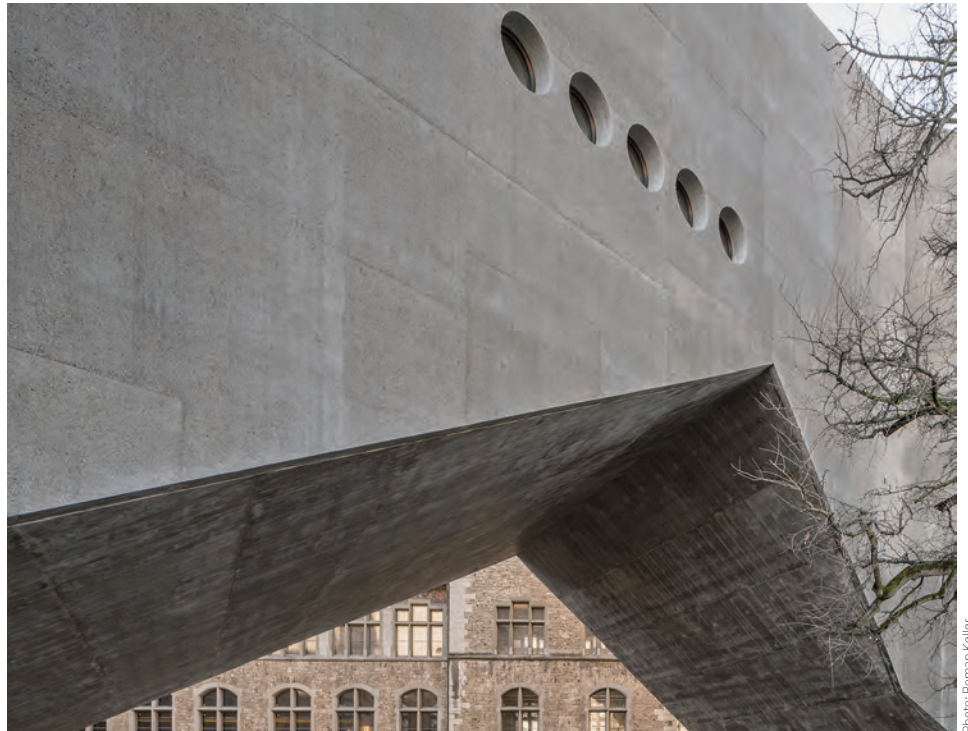
ABOVE Christ & Gantenbein's extension to the Swiss National Museum in Zurich. The external concrete contains a proportion of fly ash as a cement replacement, which darkened the tone and reduced the water content
