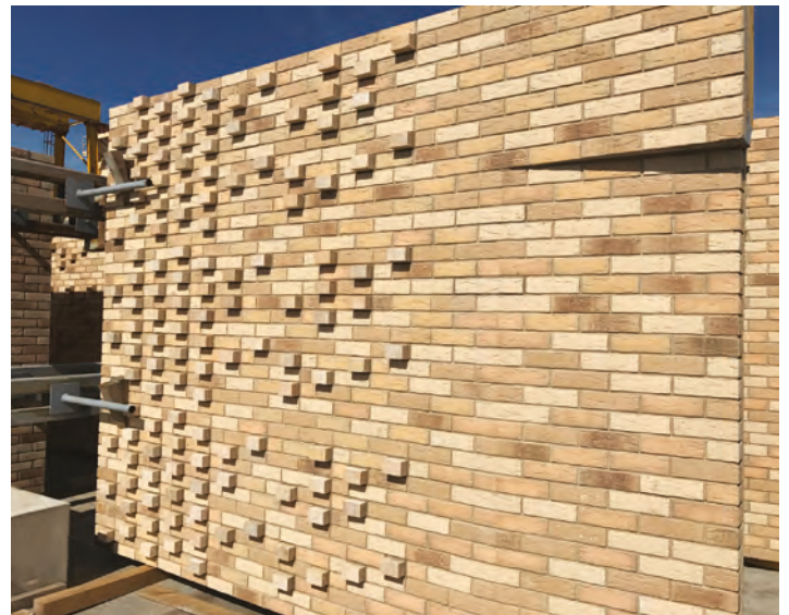
ABOVE The Lansdowne, a 16-storey apartment building in Birmingham designed by SRC and Building Design Group. The precast cladding panels, supplied by FP McCann, are 410mm thick and comprise an insulation layer between two concrete faces with an outer 80mm-thick facade consisting of a detailed buff brick design
