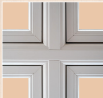
162mm Sash / Mullion / Sash sightlines with Arrissed Joints Mimicking Traditional Timber Joinery
