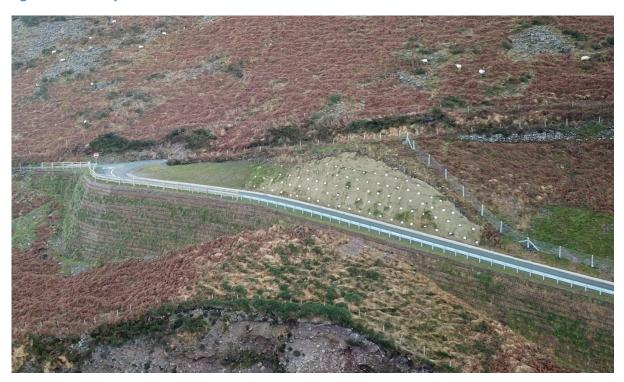
Figure 6 - Soil nailing at cut section below existing road
