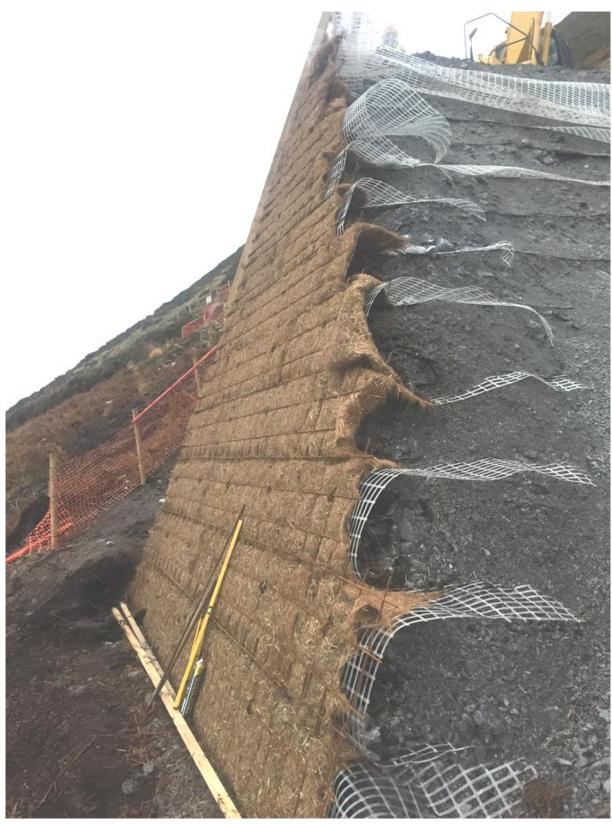
Figure 7 - Embankment under construction
