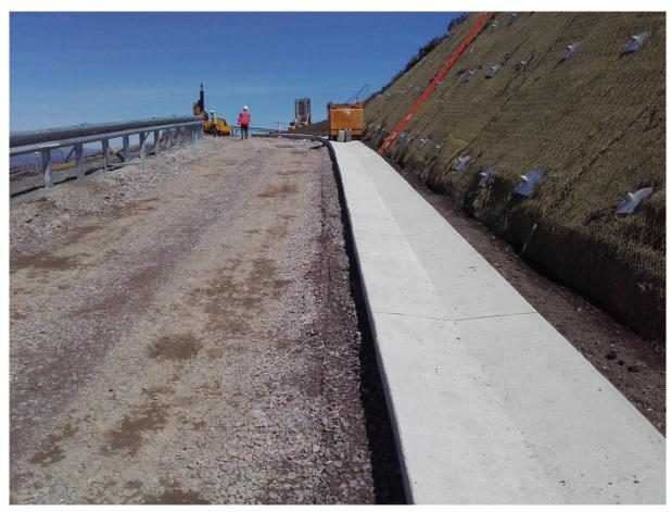
Figure 9 - Drainage channel
