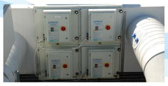
$4\ \mbox{ESP}$  Units Stacked in modular formation with a double pass
