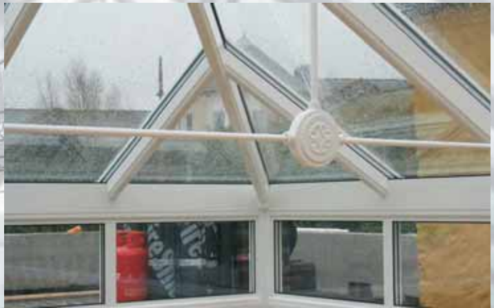
3 Way Tie Bar to stop trust loads
