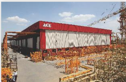
Tower Crane Plant
