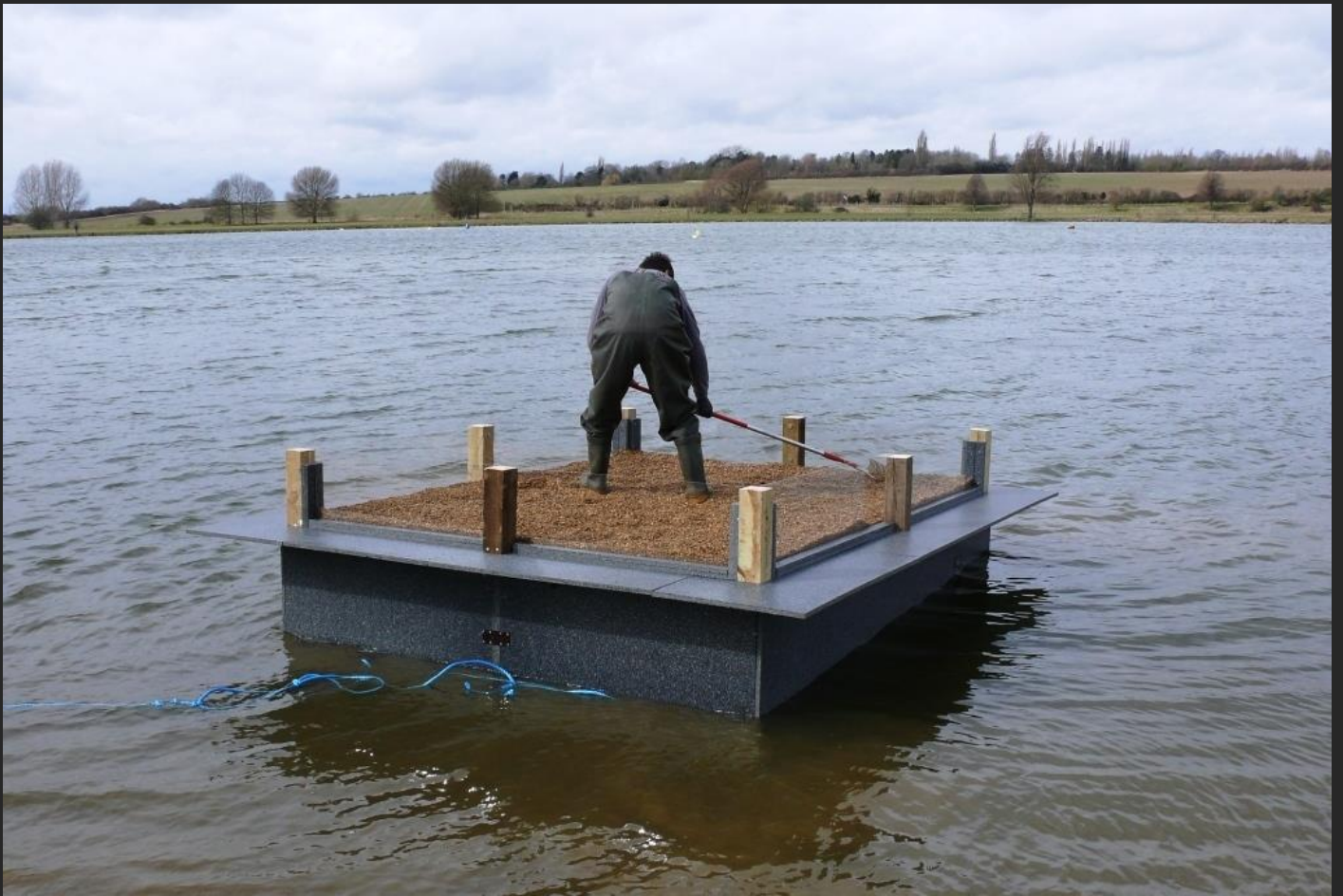
2 tern nesting rafts designed to be mink and otter proof, with Perspex sides for 'birders' – installation at the Nene Park Trust Peterborough March 2013. Units are unsinkable due to their internal fill. They are fabricated at our Isle of Wight Factory from 85% recycled materials.
