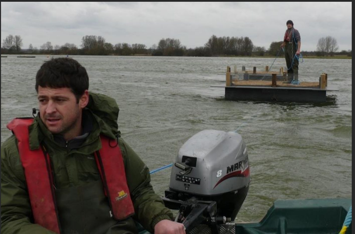
2 tern nesting rafts designed to be mink and otter proof, with Perspex sides for 'birders' – installation at the Nene Park Trust Peterborough March 2013. Units are unsinkable due to their internal fill. They are fabricated at our Isle of Wight Factory from 85% recycled materials.
