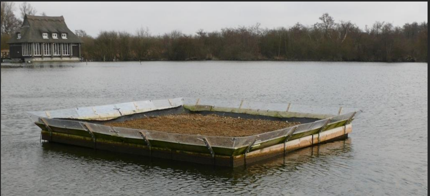
A Trial 'Concept' Tern Raft Installed 'free of charge' on Ranworth Broad – Norfolk Wildlife Trust
