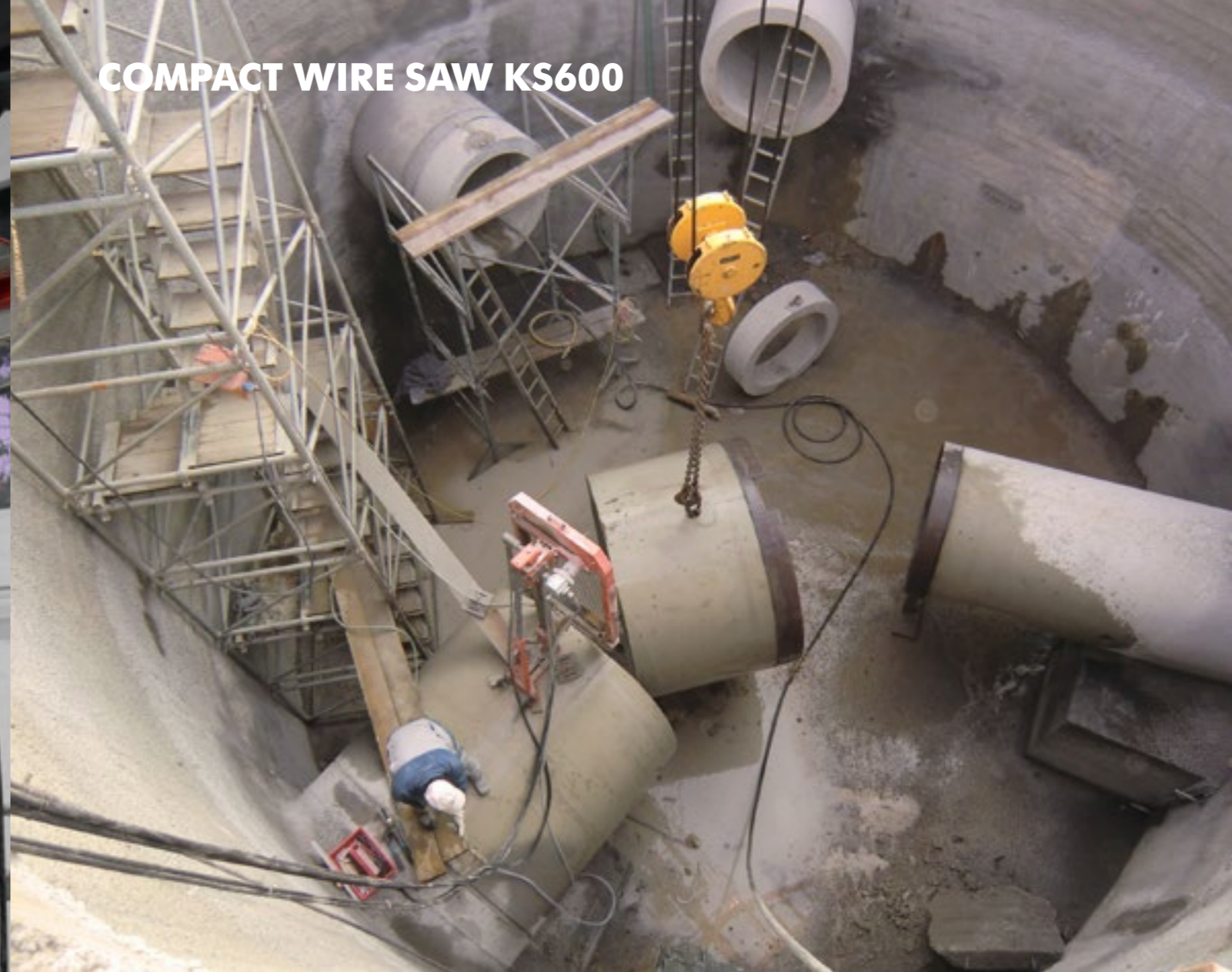
Efficient and quick cutting of CONCRETE PIPES directly in the central shaft. GÖLZ modular system allows short setup times and easy transport on and to the jobsite.
