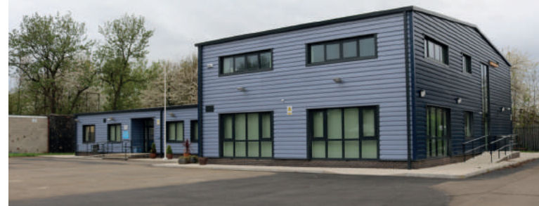
(Top) Hinckley Joint Cadet Centre (Bottom) 126 (City of Derby) Sqn HQ
