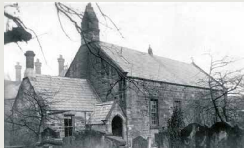
The Chapel of Ease, 1924, just prior to demolition.
