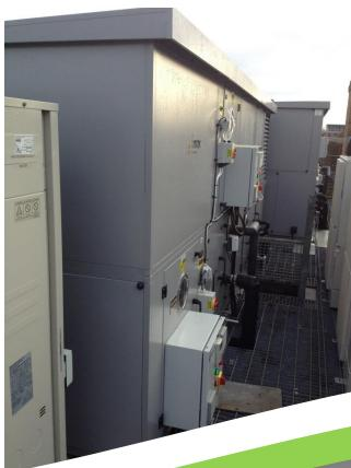
Constant Air Systems Ltd acted as principal contractor where we completed the removal of the existing air handling plant and installed new plant at roof level, connecting to the existing air distribution for the museum.
