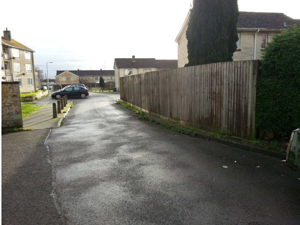
Image 01: The view along the access road into the garage site, facing back towards King Lea Avenue and Long Close Avenue.
