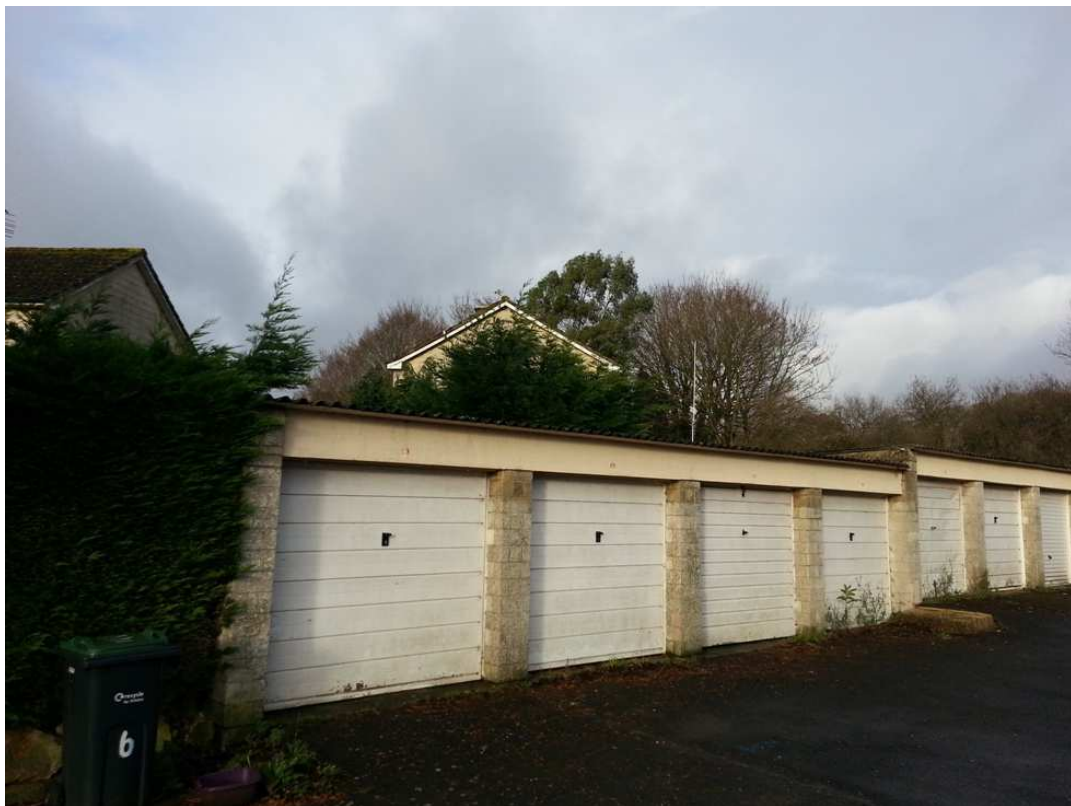
Image 05: Turning to the right, the larger garage block stretches north toward the open field beyond.
