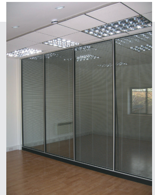
Full height glazing with blinds
