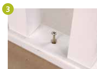
3 Unscrew the floor rail.
