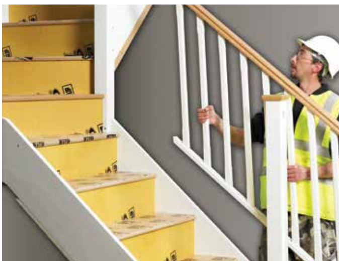
Demountable balustrade unclipped and removed
