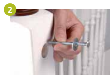
2 Unscrew and remove the bolt holding the handrail and keep safely.
