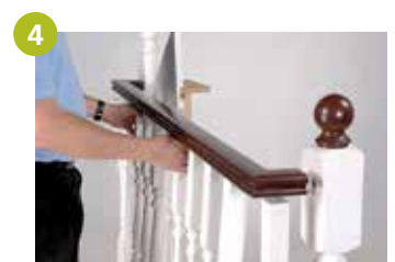
4 Once all the fittings have been removed, the section of assembled balustrade is simply lifted off.
