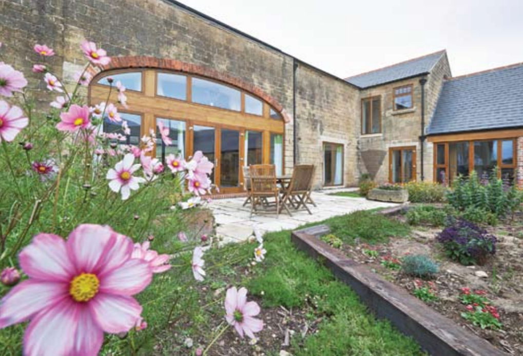
Barn conversion Nottingham
