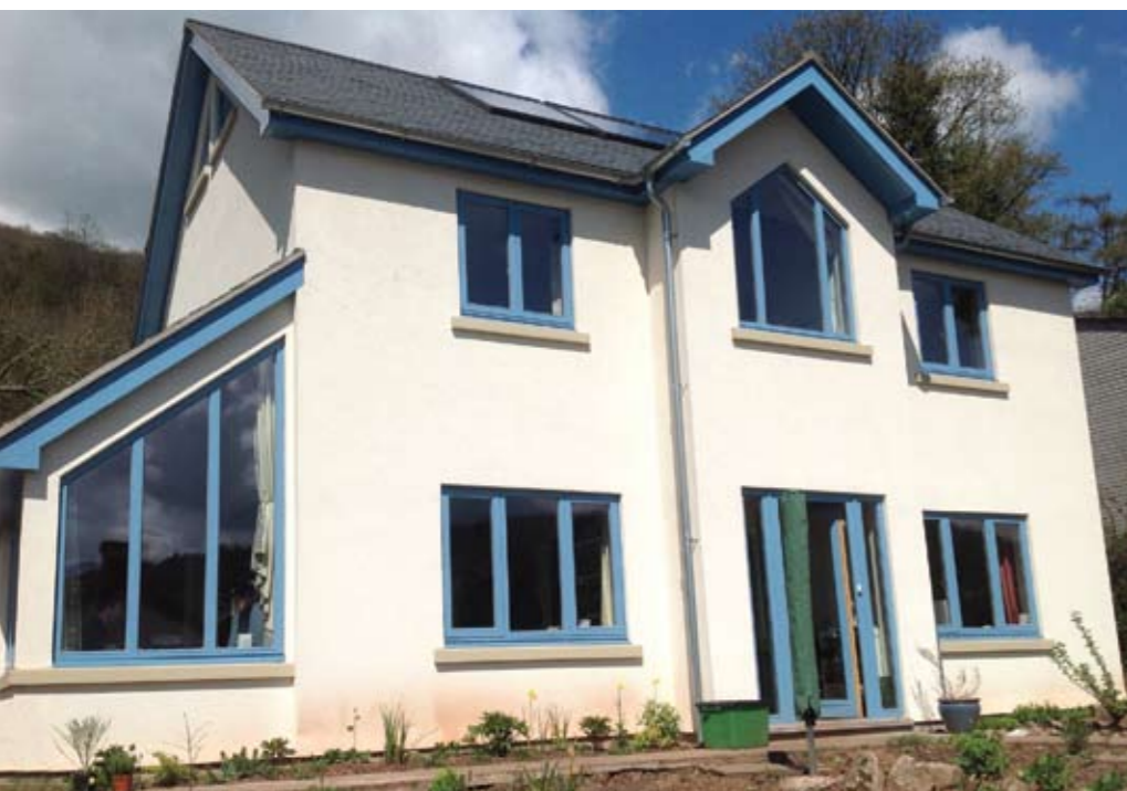
Newbuild house Monmouthshire
