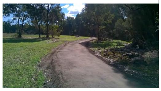
Figure 3: Bitumen Stabilised Limestone access track installed around 1.5km of the reserve
