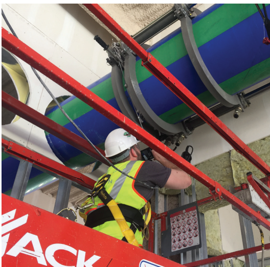
The McElroy Acrobat™ 630 fusion machine was designed to enable fusion of large-diameter PP-R pipe in tight spaces.
