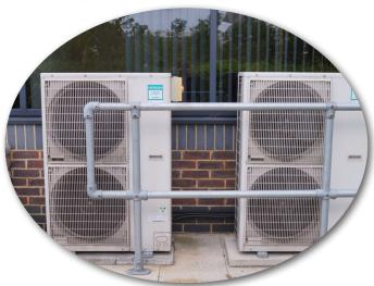
Air source heat pumps are a very efficient way of providing heat for your hot water or heating system by extracting heat from the air outside and transferring it into a building. They work in a similar way to refrigerators, but in reverse. They are similar in appearance to air-conditioning units.
