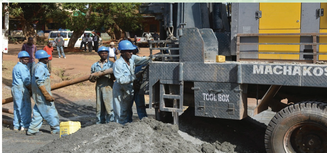
Drilling of a borehole in Machakos County
