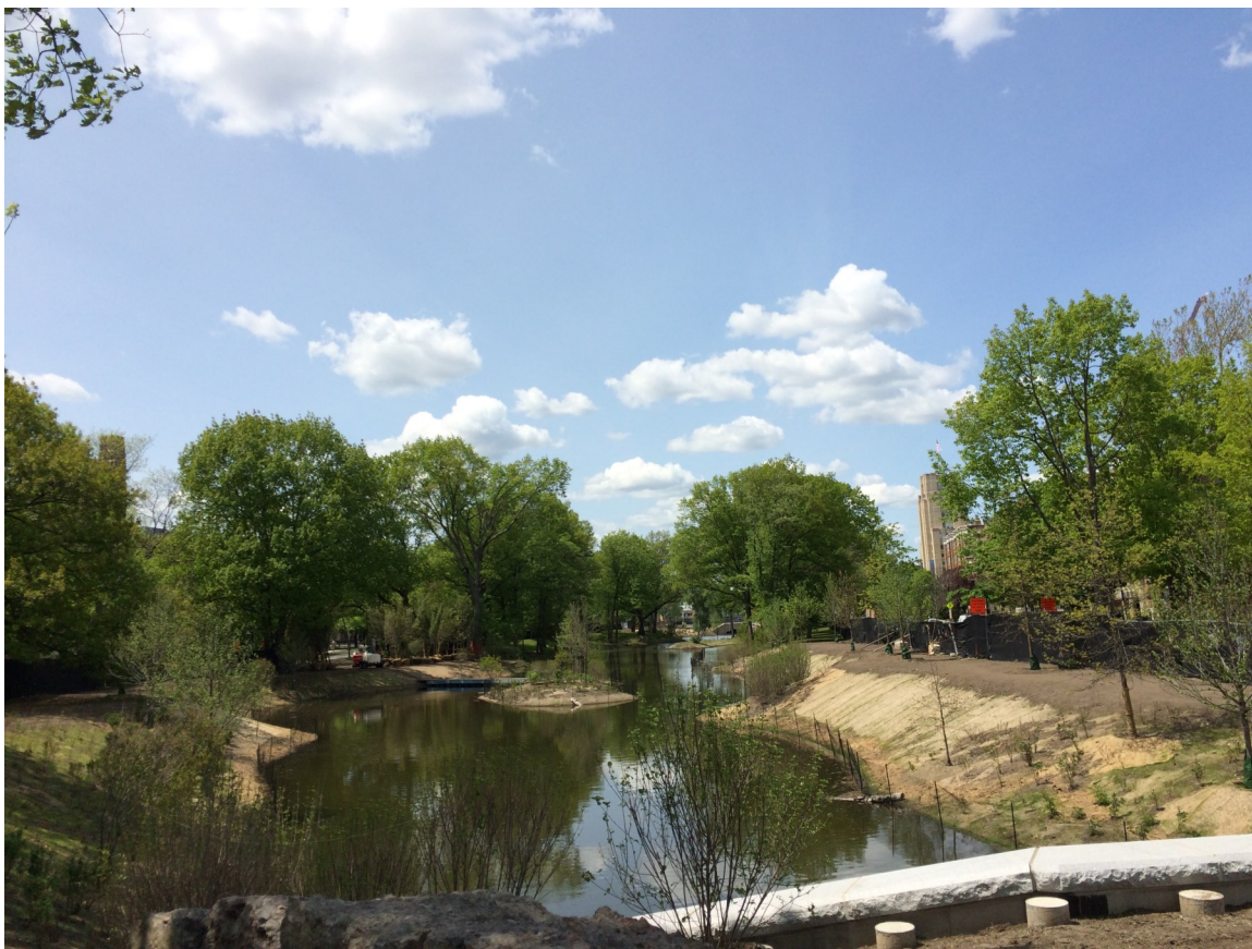
Muddy River Restoration Project new plantings and daylighted river
