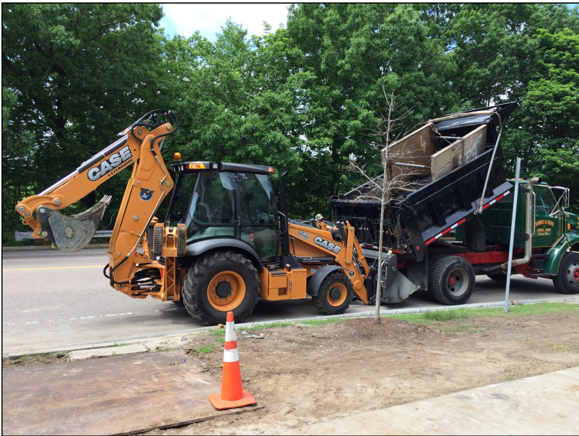
Boston Water and Sewer Commission Water Main Work on The Riverway
