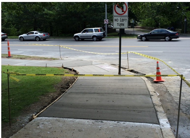
Sidewalk ramp reconstruction along the Riverway
