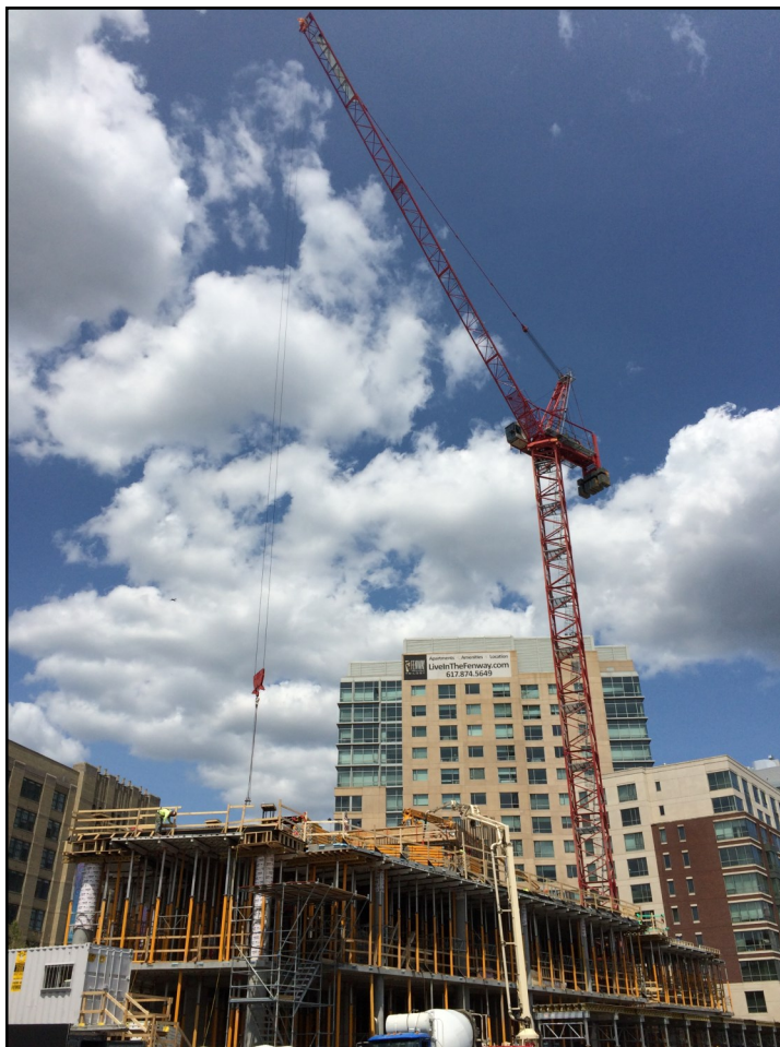
Tower Crane at the Pierce Project
