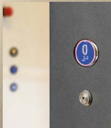
5 ENABLING KEY at landing
