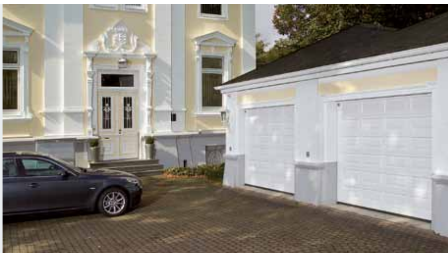
Panelled in Hemlock, wood preservative in Limestone white
