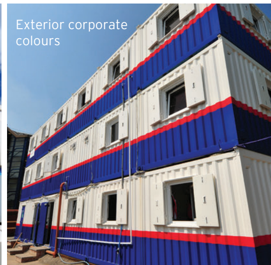
Doubled glazing and exterior anti-vandal shutters. Exterior staircase with linkway
