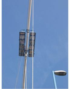
In order to install the manifolds required by the main cable dehumidifying system a pair of ALPS Steel Truss Frame access platforms were assembled and installed to the required location, these moved as required from location to location.
