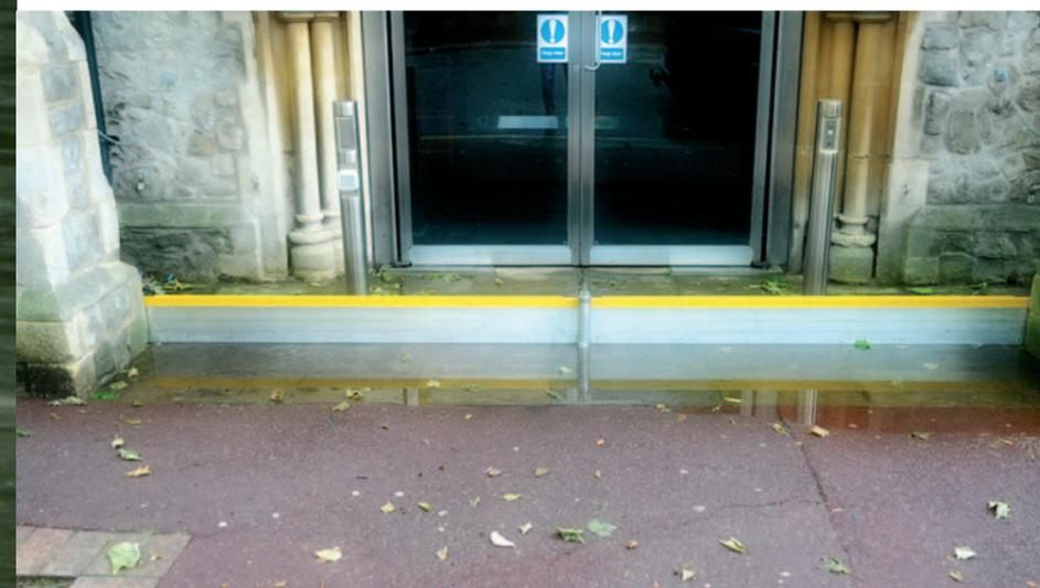
Suitable for installation on both residential and commercial property, Nautilus® 200 makes use of two permanently-fixed vertical side channels fitted either side of the opening to be protected, along with pre-installed unobtrusive ground fixtures to allow the Patented Twist and Lock post system (Patent No. 2371068) to be put in place.
