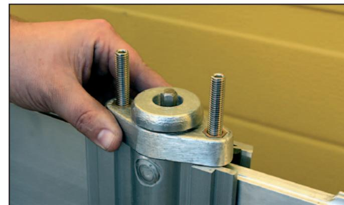
**1** Secure the flood board(s) by inserting the vertical side channel compression blocks (slotted into the top of each channel).
