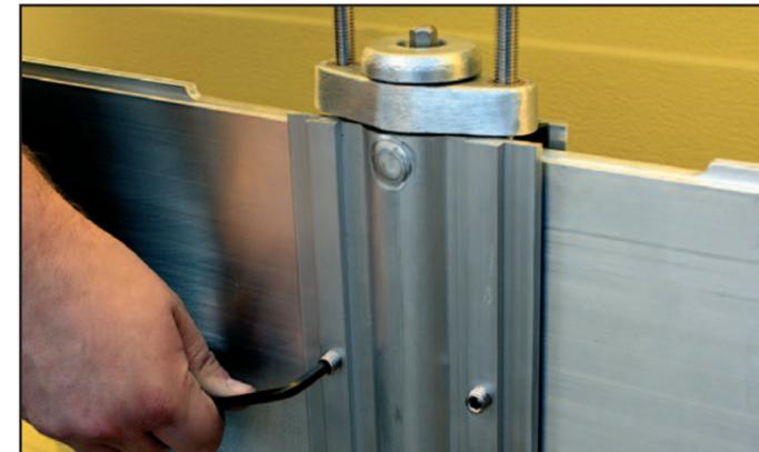
**8** Using the 5mm Allen Key, turn each 10mm grub screw, clockwise, in the top compression blocks, one full turn (360 degrees).
