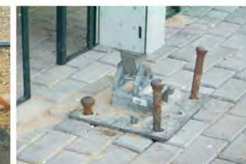
● Steel Ground Anchor Fixation
