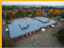
LIQUID APPLIED ROOFING
