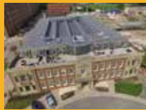
SINGLE PLY ROOFING
