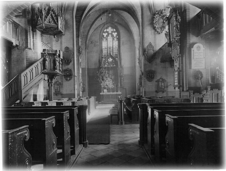
Inside St. Barbara's Lutheran Church
