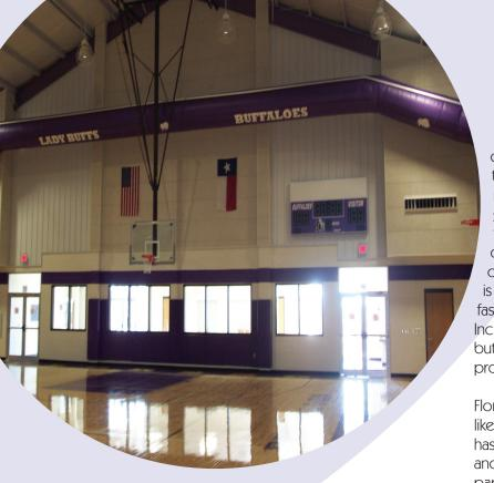
While Fromberg likes the streamlined aesthetics, Kent specifies fabric duct because of cost-saving benefits as well as performance characteristics. Performance tests prove that fabric duct disperses air more evenly and efficiently than metal duct/register configurations. Thus it fit Kent's energy efficient HVAC system design that uses energy recovery to treat outside air and save Florence over 50 percent in air conditioning operating costs versus conventional DX equipment designs.
