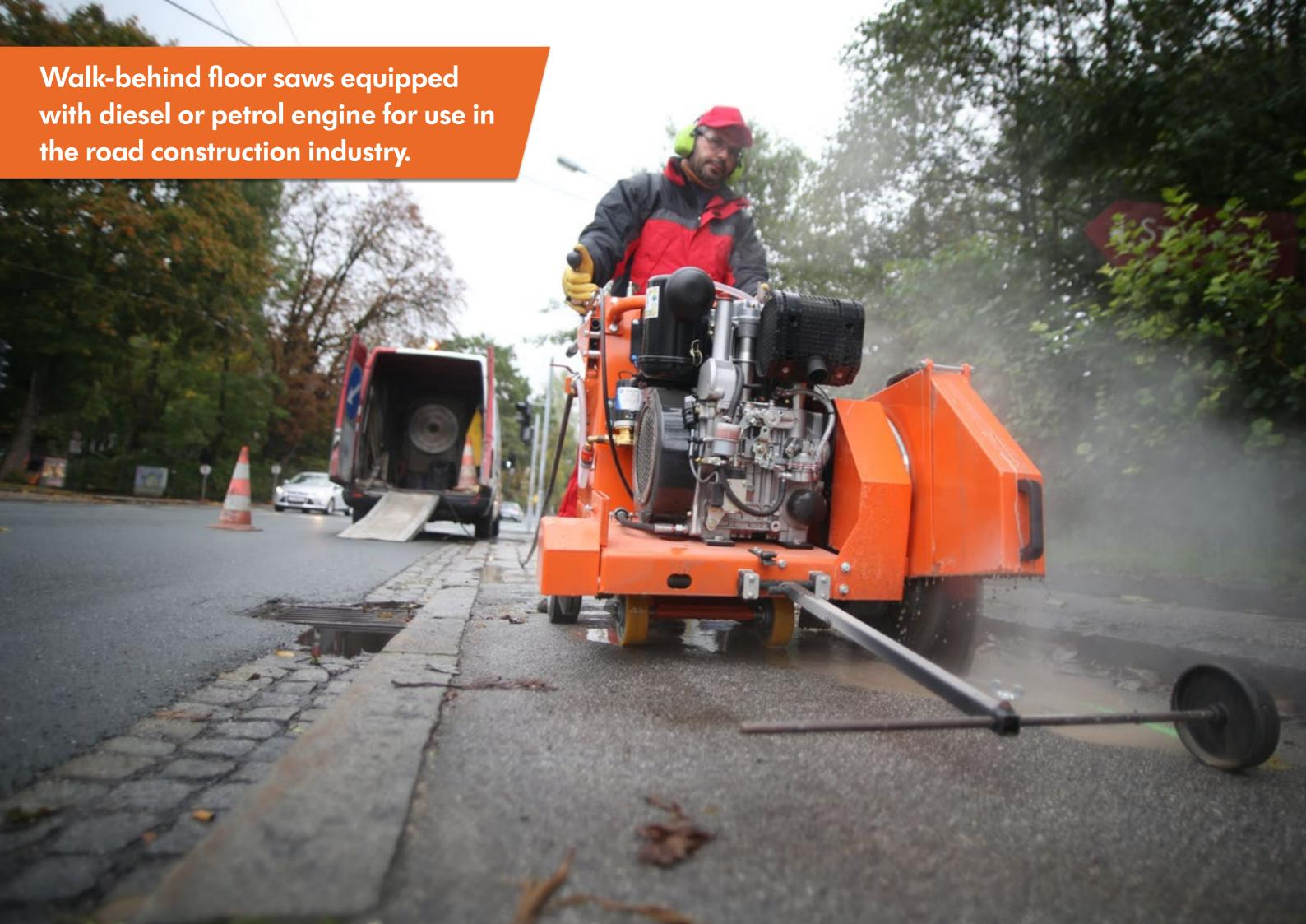
FS190 Floor Saw Floor Saw FS190
