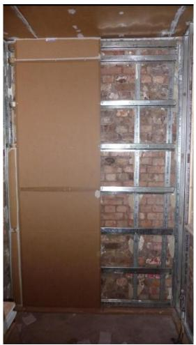
Resilient Bars are then installed horizontally on to the C studs at 600mm centres. The bottom bar should be positioned close to the floor and the top bar should be close to the ceiling but they must NOT touch the floor, the ceiling or the surrounding walls as this will cause noise to transfer into these structures.
