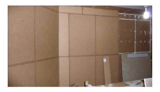
This wall has been completely covered in PhoneStar boards so that they are tightly butted up to the PhoneStar boards on the ceiling.
