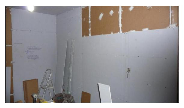
Acoustic plasterboard is then secured by screwing into the resilient bars only, using 38-42mm drywall screws. If possible use a brickwork pattern. If you are only treating the walls and not the ceiling then leave a 5mm gap all around the perimeter edges and seal this gap with permanently flexible sealant. In this case the ceilings and walls have both been upgraded to create an acoustic seal, so the plasterboard can go into the corners.
