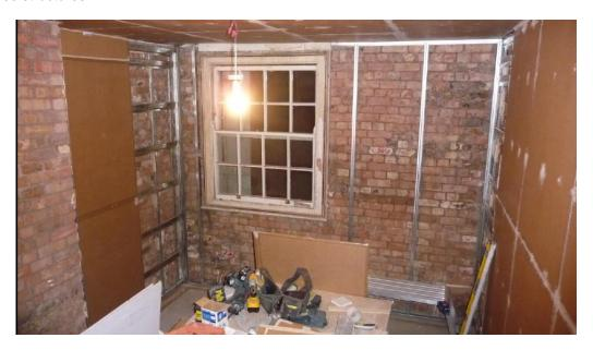
The PhoneStar boards are screwed to the resilient bars only using 25mm drywall screws. These screws must NOT penetrate into the wall. If possible fix the boards in a brickwork formation. Butt the boards tightly up to each other and to the perimeter walls, floor and ceiling. Ensure the PhoneStar board edges are sealed with PhoneStar Eco-tape after cutting to minimise sand spillage.
