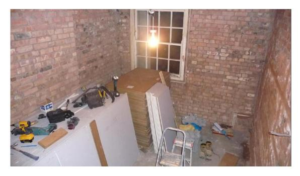
These walls have been stripped back to the bare bricks. Although this is not necessary it allows the installer to seal any gaps in the mortar or around electric wiring as well as all the perimeter edges. In addition it saves living space.
