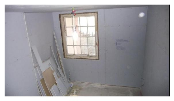
This shows the finished walls and ceiling, apart from around the window. Please note the gap at the very bottom of the plasterboard at floor level. This should be sealed with permanently flexible sealant. The plasterboard joints and screw heads are then sealed as normal. The skirting board should have a very small gap between it and the floor to reduce the risk of flanking sound.
