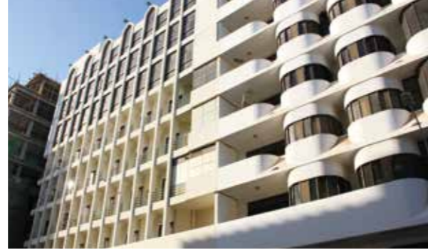
Trading Building Air Cooled Screw Chiller Oman
