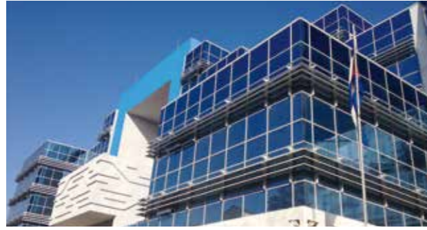
CECMED National Drug Laboratory Water-cooled Screw Chiller Hydronic Air Handling Unit Fan Coil Unit Cuba
