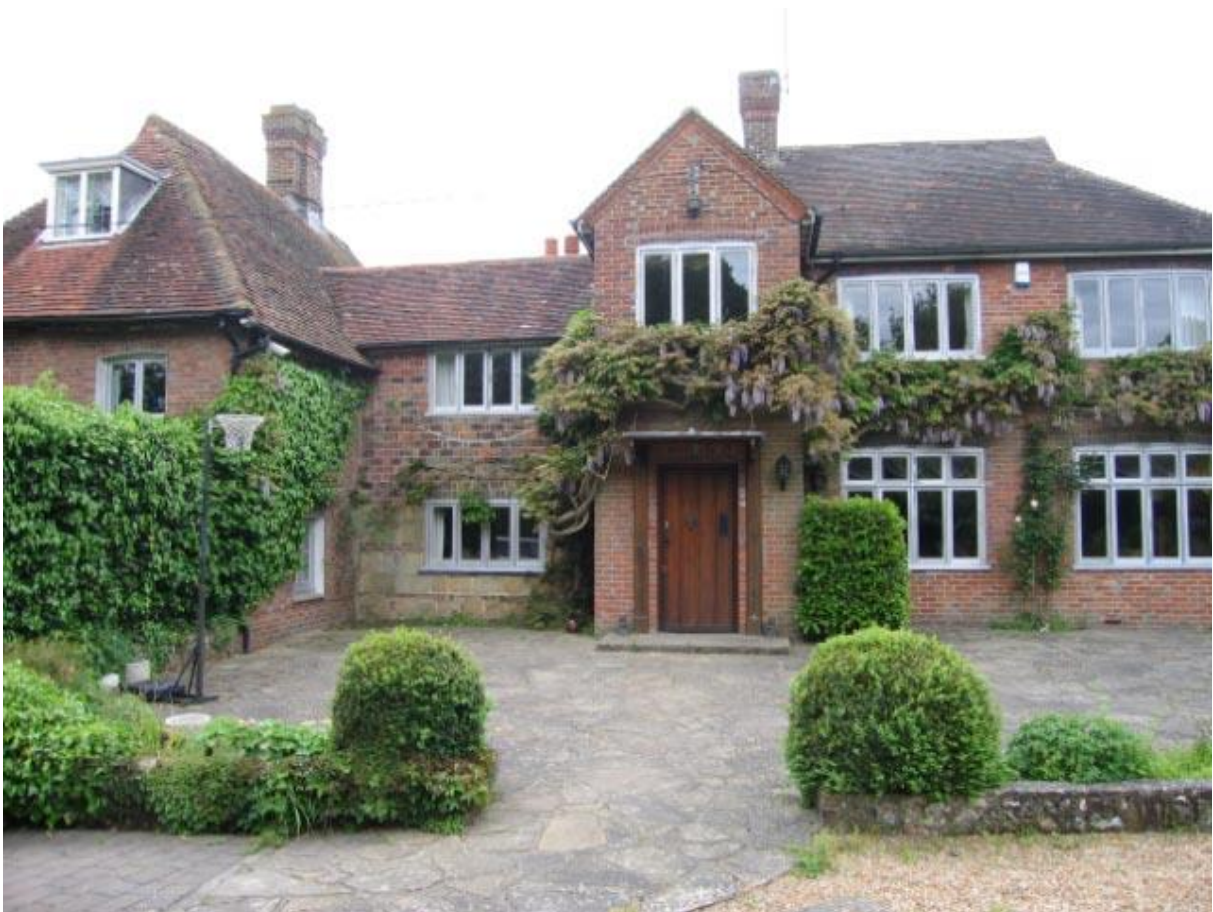
Replacement windows in a listed property in Wivelsfield Green
