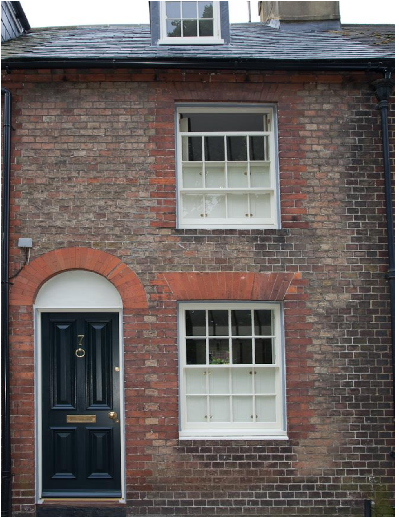
Replacement of vertical sliding sash box windows in a terraced property in Lewes, East Sussex.
