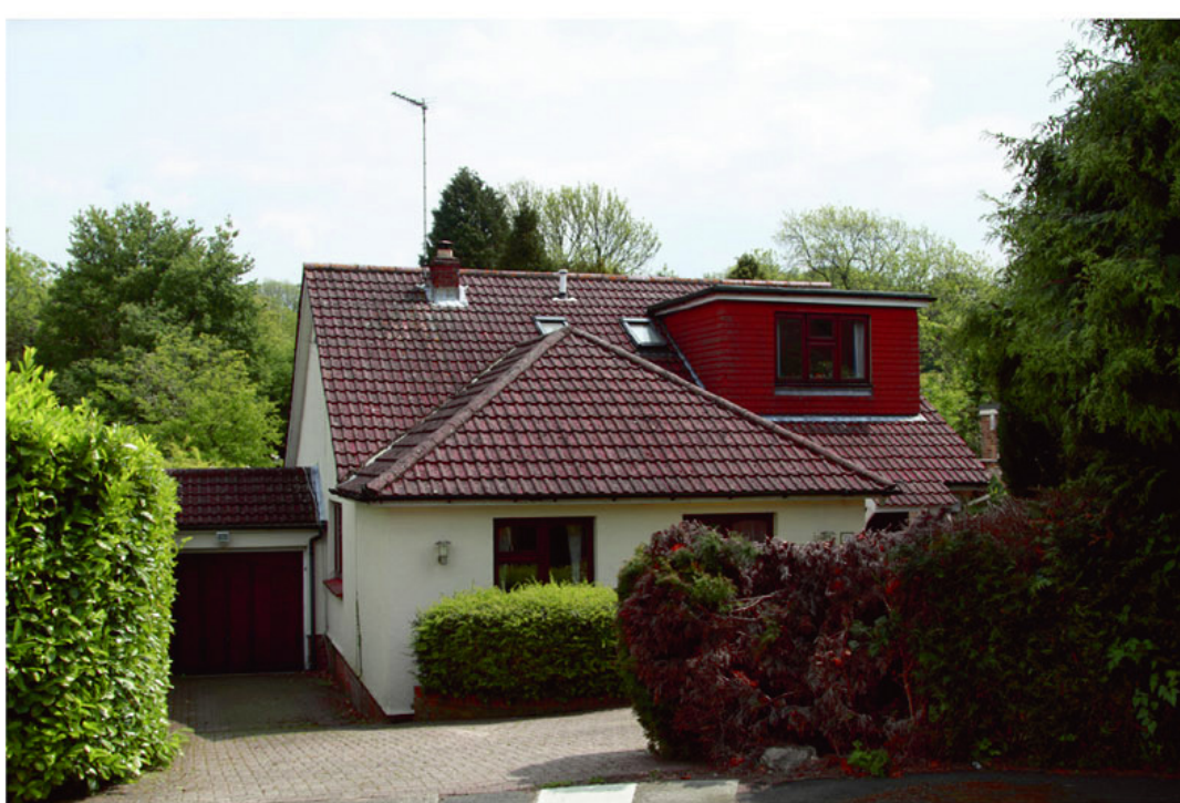
View from the road at ground level
