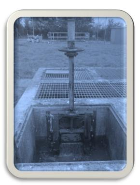
The equipment used was the HVL-VR Valve Operation System. This tooling was able to engage with the valve and release the valves from their seized position.
