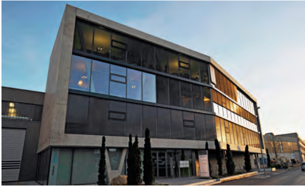
Head Office, Brugg, Switzerland
