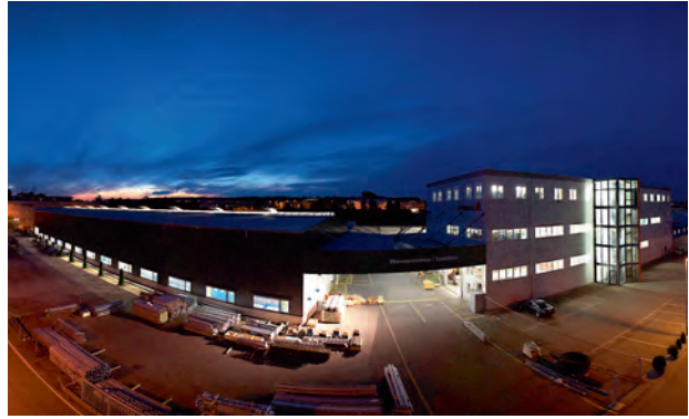
Geobrudd AG, Romanshorn, Switzerland
