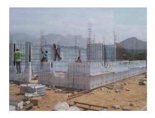
The combination of a modern formwork mould system and lightweight cellular concrete is ideal for fast construction of good quality, affordable houses.
