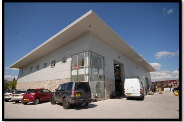
The front high side has two 3m wide x 6m high opening and one end has one 3m wide x 6m high opening with PFC door posts. The glazing at one end is formed with PFC posts.
