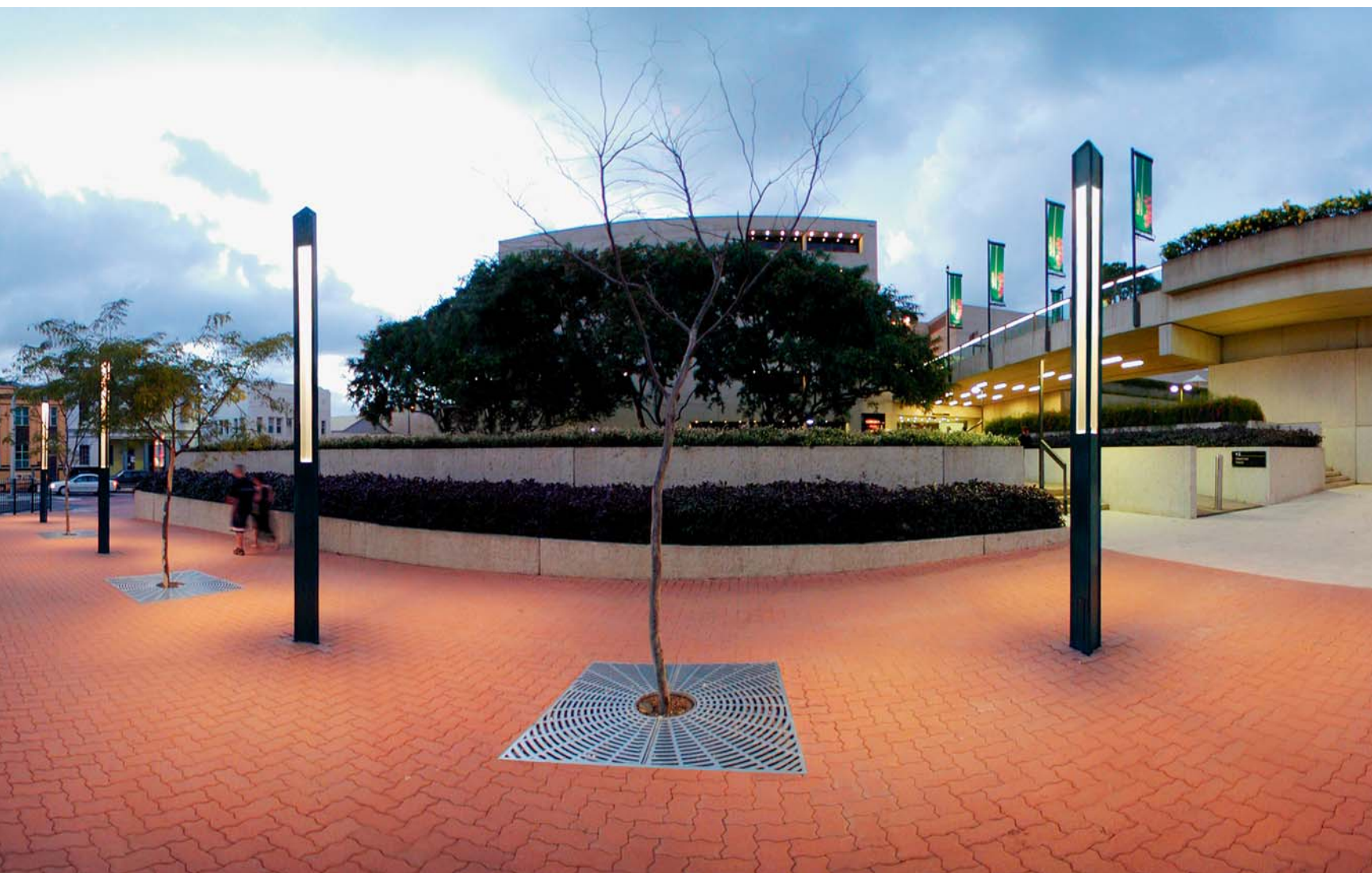
South Eastern Busway. Cultural Centre Station. Brisbane (AUS)
